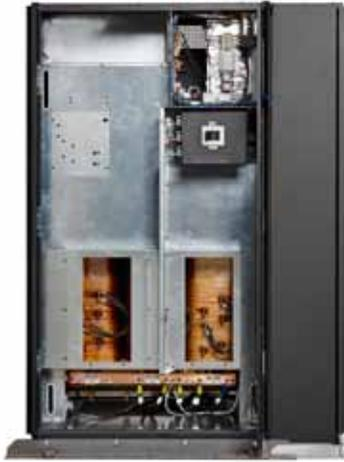
Front Access PDU with transformer access covers removed
