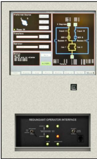
WaveStar display and redundant operator interface
