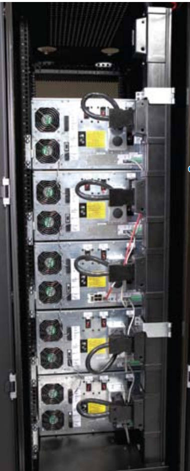
The BladeUPS Parallel Bar easily connects up to six modules in parallel.
